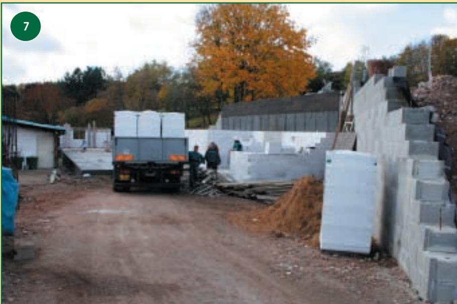
Essential for the new house was a new retaining wall; almost five metres high, it allowed the building being positioned closer to the service road and the house being set into the existing slope above the former zebra
